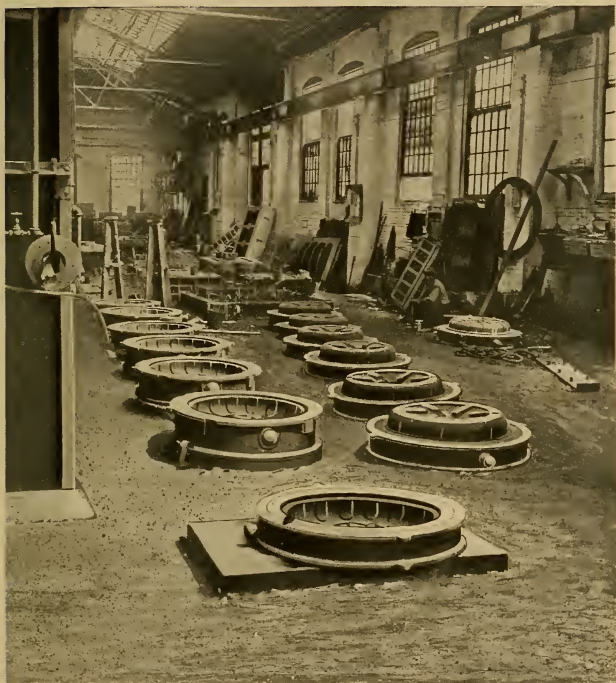
Fig. 76. A floor of Generator End Frame Moulds made on the Plain Jolt Machine shown in the foreground, at the plant of THE WESTINGHOUSE ELECTRIC & MFG. CO. Cleveland, Ohio, U. S. A.
